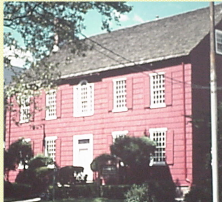
Restored Boudinot Mansion
