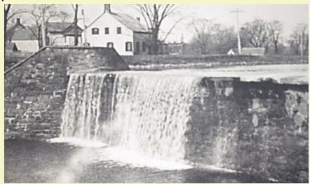
At the same time the old dam was re-enforced with a massive concrete casting, and a new iron and concrete bridge replaced the old iron bridge over the Elizabeth River at Trotter's Lane, just to the left off the picture.
